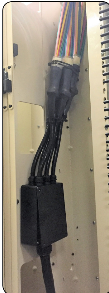
Kits During Installation
