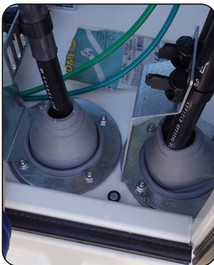
Use customer supplied sealant to seal entry cones
