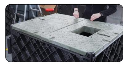
7. Fully tighten the bolts securing the lid to the vault.
