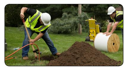
Whether pre-connectorized or not, here are a couple quick tips to use when installing pushable fiber into the microduct. These techniques have been used to install single fiber, connectorized fiber and multi-fiber assemblies at distances in excess of 500 feet.
