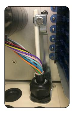
19. Tighten the dome nut on the sealcon securely, being careful not to damage the threads.
