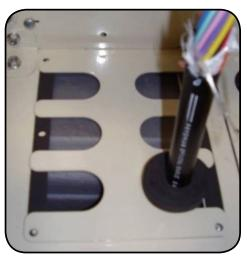
6. Feed through plate B can then be slid onto the cable followed by the cable clamp bracket. All four pieces can now be pinned together in the air by using 4 of the kit mounting bolts
