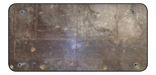
**Note:** To not degrade the anchor's installed performance, any unused anchor holes (or other nearby holes) in the concrete within 3" must be filled with an epoxy filler (pour stone) or equivalent. Filled holes must be fully cured before anchors are installed and torqued.
