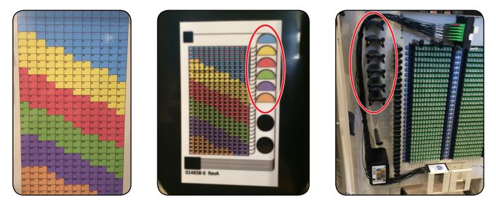
8. Splitters can only be routed and deployed on their respective side of the insert. Each half of the PON Insert holds (9) splitters. There are more feeder ports than (9), allowing for pass through/express ports if needed.
