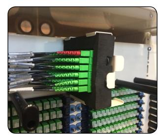
7. In the bottom left and right corner of the panel, you will find a routing guide to help determine the proper spool to route the splitter legs over when deploying. You will notice that the provided desi-card has corresponding color coded squares. Simply route the cable over the spool associated with the color of the port you intend to activate and the slack will be properly addressed.
