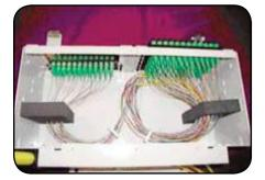
2. Before bringing in the fiber, install the included self-adhesive foam separators and cable management clips. Trim the foam separators to the correct height for the panel that is being installed.
