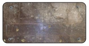
Using a 5/8" masonry bit, drill the four required holes to a minimum depth of 50 mm (approx. 2").
