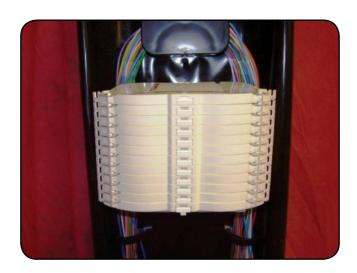
**Note:** If more than 6 trays are used, you will not be able to hinge the entire stack to access lower splices. Although the bracket will accommodate 12 trays, Clearfield recommends only using 6 trays for 72 splices. Trays can be added by sliding the new tray onto the hinge pins and then folding it down to snap the tray in place.
