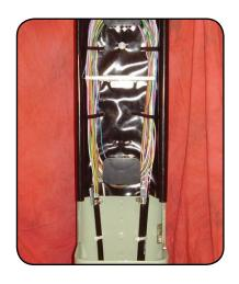
The excess buffer tube should then be routed loosely around the radius limiters provided and then secured loosely with the Velcro management that is installed in the pedestal.
