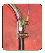
3M 4460-D Bonding clamp installed
