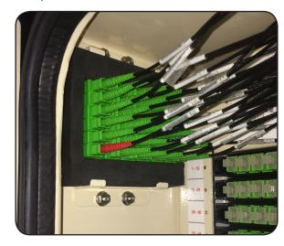
Two splitters: Remove foam cradles from staging plates, and place foam strips. Insert staging plates vertically into staging area at top of cabinet.
