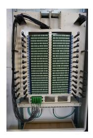
the staging plate storage area and deploy subscriber circuits from there. Due to the highly configurable design of the FieldSmart 576-port FAC Fiber Insert, splitters and WDM components can also be deployed in the Clearview Cassette. For optimum flexibility and crush resistance, ruggedized cabling is used throughout.
