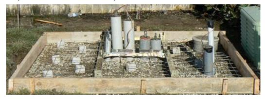
**Note:** The template's mounting studs should protrude approximately 2 inches above the form.
