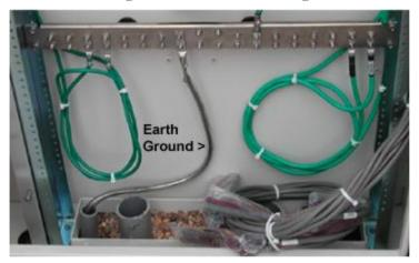
**6.** Re-connect the nuts to the ground terminal studs and tighten to 26 inch-lbs. of torque.
