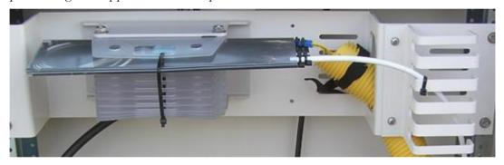
**4.** Route the fiber pigtails from the splice tray through the fiber routing conduit to the distribution system or the equipment.
