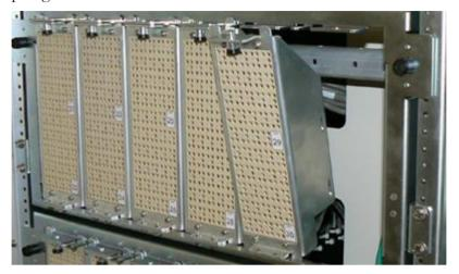
c. Fasten the protection block to the mounting frame using two supplied screws.
