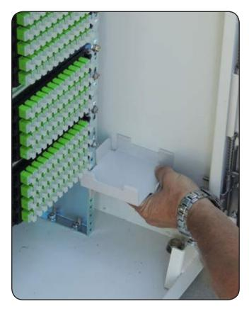
**d.** While holding the bracket against the rack, install the mounting screw to secure the staging area to the rack. Tighten the screws to 45 in. lbs. of torque.
