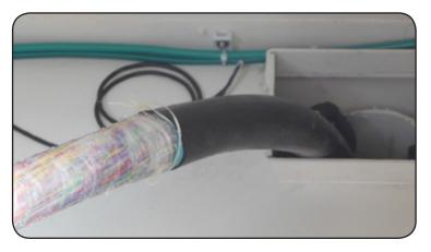
**Step 4:** Ground the OSP cable sheath to the cabinet's main ground bar or EXM's subground bar as follows:
