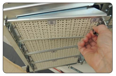
**a.** Insert the tabs on the left side of the block into the slots on the mounting frame.
