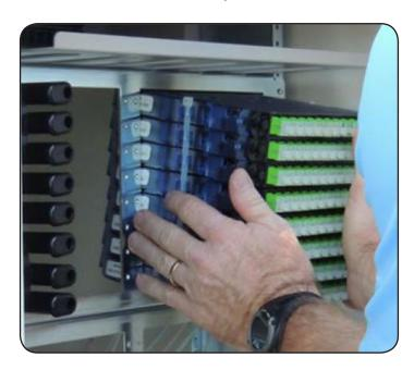
c. Align the mounting holes on fiber termination assembly with the counterpart holes on the frame.
