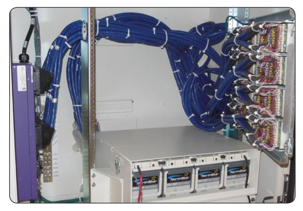
**Step 6:** Apply line identification labels over the protection block's dead pair positions (25, 50).
