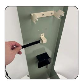
Insert the splice trays into the splice treay mounting bracket as needed. Splice trays must enter the bracket while in a horizontal position, then allowed to swing downwards. Splice trays cannot be pulled out of the bracket while in a vertical position.
