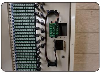
4. Utilize the routing diagram shown here to connect splitter legs. Remove the connectors from the staging plate, route the fiber over the radius finger in the first row that best takes up the amount of slack needed, and between the two radius fingers in the second row that most closely align with the intended port.
