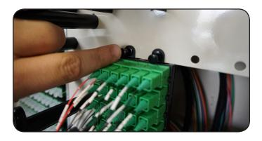
2. Install the body of the splitter into the splitter cage by hooking the top finger of the splitter underneath the top rod. Then swing the bottom of the splitter body down, engaging the clip with the lower rod of the splitter cage. Press hard until it clicks into place.
