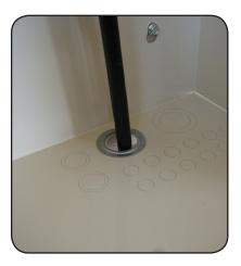
5. Select the compression fitting grommet size that most nearly fits the cable to be installed. Grommet kits must be ordered separately, contact your sales rep.
