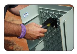
The bolt of the top mounted bracket can then be slid into the gap in the mounting bracket.
