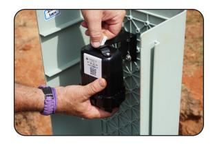
4. Secure the SeeChange terminal in place by tightening the wing nut on the bolt.
