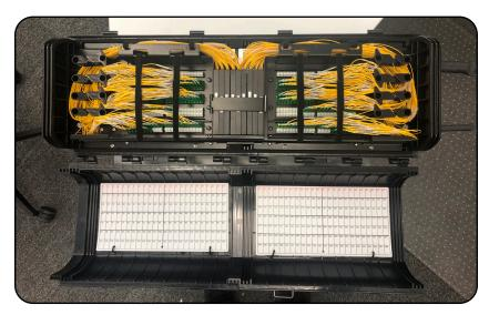
One half of the Aerial FDH's ports are shown here. The top row will consist of feeder ports, and the remaining rows are distribution. The blank spot in the center of the bottom is the staging area, where the splitter's staging plate will be installed and which will hold uninstalled splitter legs.
